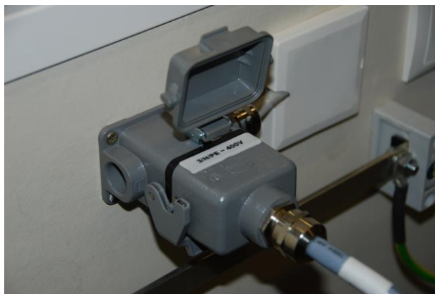
Fig. 42: Connection variant 2: fixed connection with coded heavy duty connector
